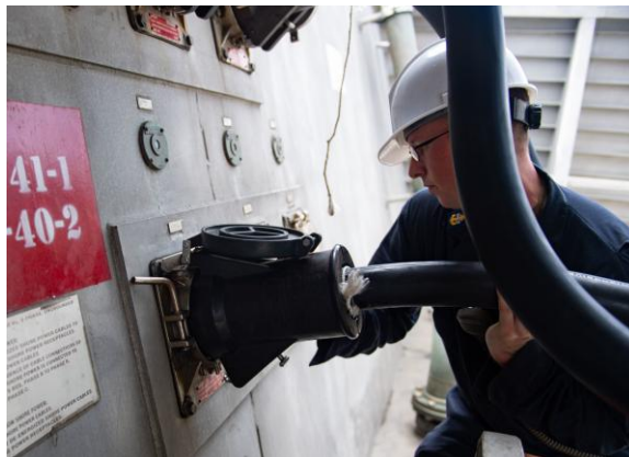
Figure 8: Shore Power Connection on USS Little Rock (LCS 9) (US Navy photo)
