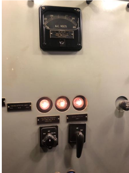
Figure 9: Ground detection lamps on USS Slater (DE 766) (photo by Norbert Doerry)
