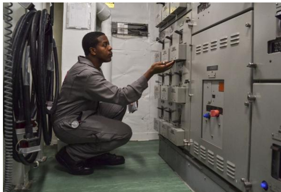
Figure 2: Load center on USS Cole (DDG 67) (US Navy photo)
